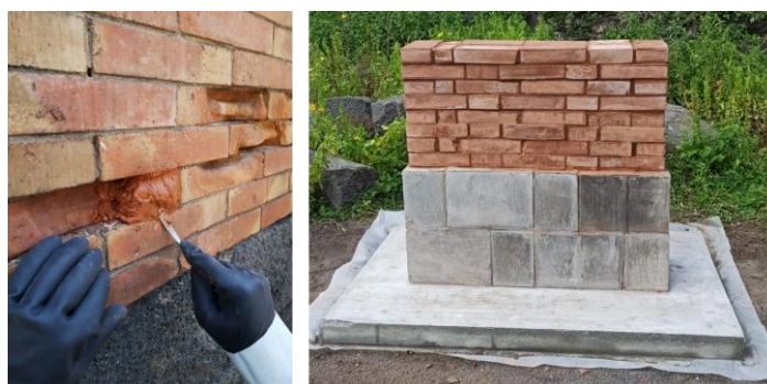
Fig. 1 – Ceramic-based geopolymeric mortar during in situ application (left) and a totally green masonry prototype (right), both exposed at the Odéon in Catania.
